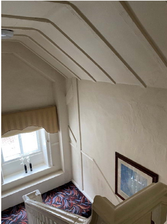
2 nd floor landing – walls and ceiling to be lined / painted with fire rated material by Envirograf.
